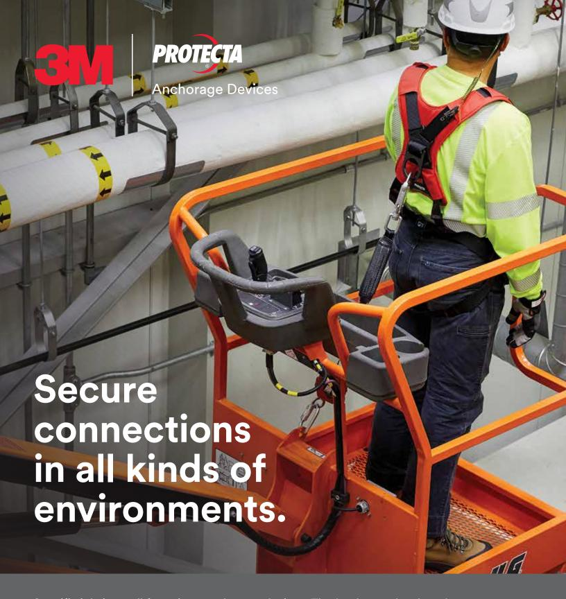
Specific jobsites call for unique anchorage devices. That's why we developed a complete line, all rigorously tested to meet OSHA and ANSI standards and help ensure strength. These devices support loads of 5,000 lbs. (22 kN) per worker, helping to anchor your personal fall arrest system to the main structure—whether it's concrete, wood, steel or something else.
