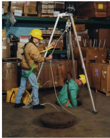
A secondary fall arrest system is recommended
